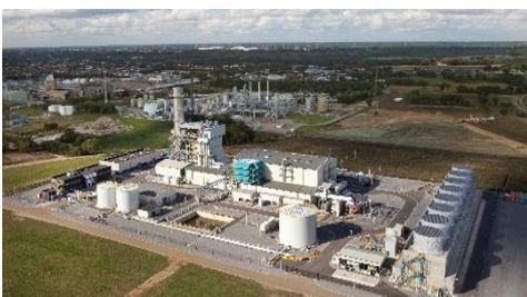
The **T-Power** segment includes the combined cycle gas turbine (CCGT) with a 425 MW capacity in Tessenderlo (Belgium).
